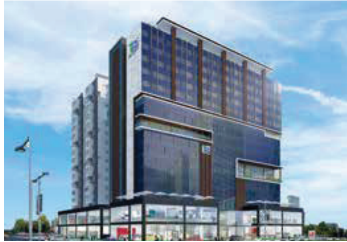
T19 Towers - Secunderabad
